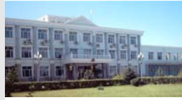
Rebuilt The office building of Changlinzi labor camp
